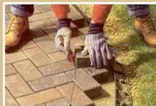
Interlock Laying
